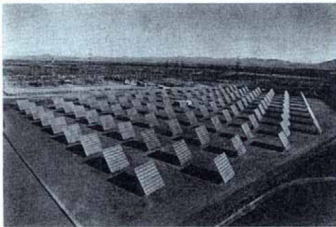
Fig 1.26 1983 AD, One million watts of P.V ARCO Solar's "Hesperia" plant in southern California. An impressive milestone in the development of large scale photo-voltaic power stations.
